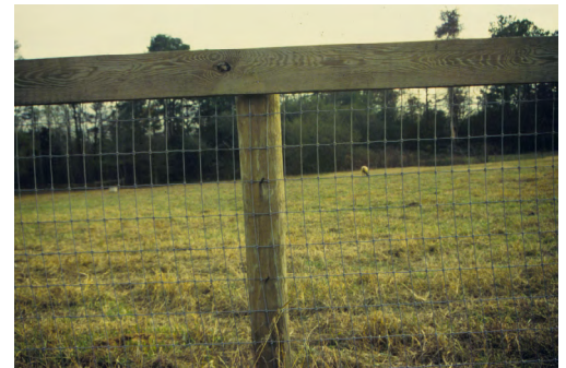
Figure 5. A top rail added to a square mesh fence prevents horses from stretching the fence wires. An electric fence wire installed on the opposite side of the post will prevent horses from rubbing on or chewing the board.
